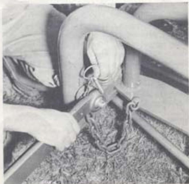
Fig. 44 Detaching Right Link
