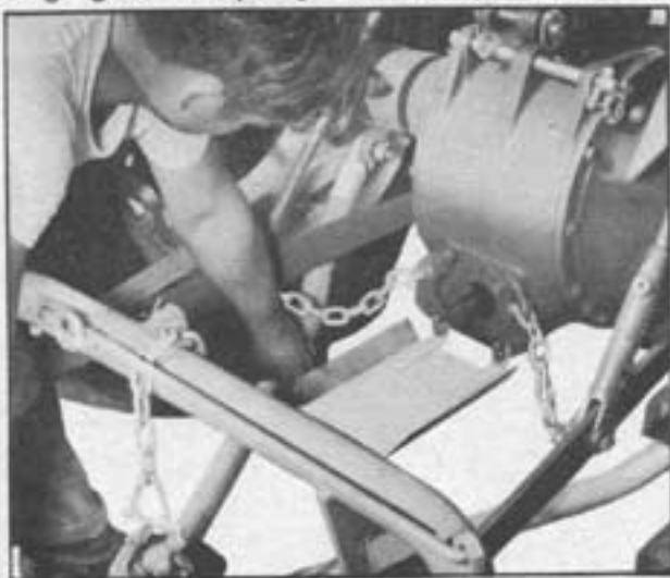
Fig. 9 Attach Left Strut
